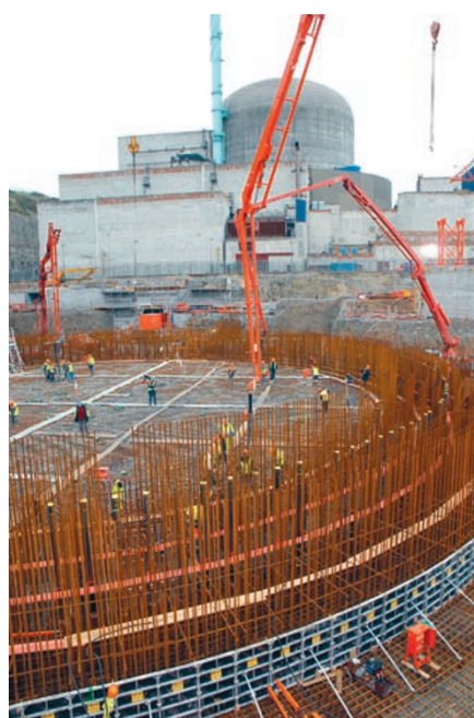
Construction of a new nuclear reactor in Flamanville, France.
