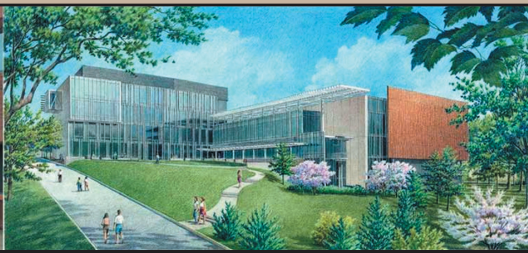
Marcus Nanotechnology Building, construction underway
