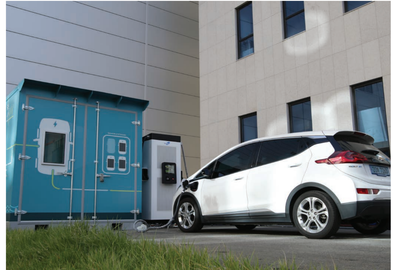
▲ A car being charged at an electric vehicle charging station installed using LGES' end-of-life EV batteries in Ochang, South Korea.
