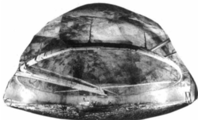
Under construction — the Super-Kamiokande observatory.
