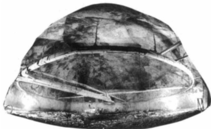
Under construction — the Super-Kamiokande observatory.
