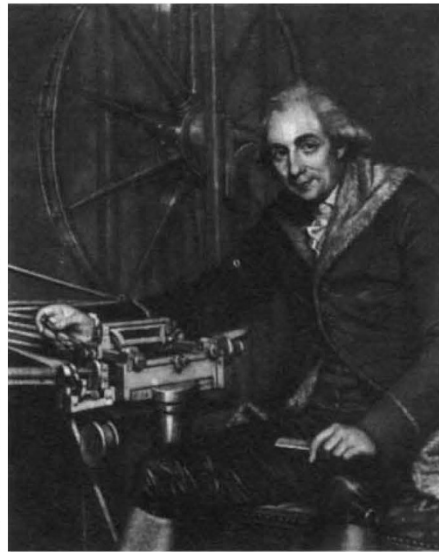
Divide and rule — Jesse Ramsden holding the old tools of his trade, but with his arm on the new dividing engine which drastically reduced the time and cost of graduating a scale.
