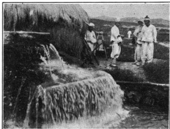
FIG. 1.—Water-actuated pestle for hulling rice, at Ching-chong-do, Korea. The bucket is shown in the act of spilling its water.
