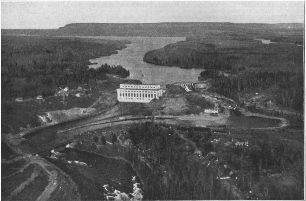
FIG. 1.—Cameron Falls development, Nipigon River, Ontario (75,000 horse power), of the Hydro-Electric Power Commission of Ontario. (By courtesy of the High Commissioner of Canada.)
