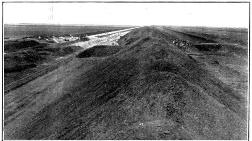
FIG. 2.—Gezira canalisation, March 10, 1925. View of main canal at Kilometer 80 from the Dam, showing a branch canal on the left, and on the right an area already developed and under cotton, and watered by pumps on the river.
