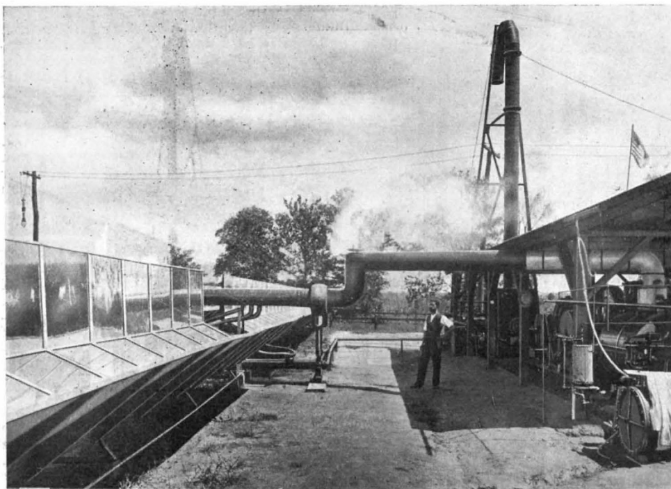
FIG. 1.—Showing one section of absorber on left, steam main and safety valve in centre, and part of engine on right.
