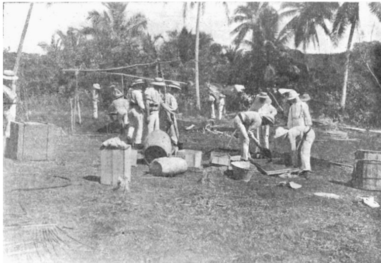
FIG. 3.—Preparing concrete for the pillars. Sand, cement, and dead coral (the last-mentioned quarried from the top of the hill) were used.
