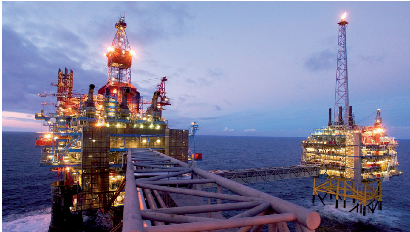
At the Sleipner field in the North Sea, waste carbon dioxide is separated from natural gas and injected into a rock formation 800 metres below the seabed.
