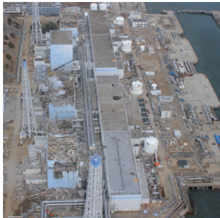
The damaged Fukushima Daiichi power plant.
