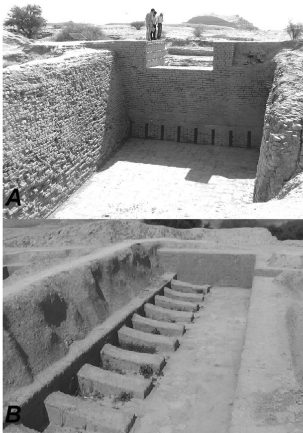
Fig. 2 The remaining of a water treatment system in “Chogha Zanbil” Complex, Khuzestan, Iran. a Front side view: Water was stored and desilted in the reservoir with a capacity of 337 \text{ m}^3 ( 10.70 \text{ m} \times 7.25 \text{ m} \times 4.35 \text{ m} ). b Back side view: The filtered water was transferred to a pond through nine conduits. When the pond was fully recharged, the filtered water was distributed by a network of canals (Adopted from Naghsh Avaran Toos Consulting Engineers Company, 2013).
