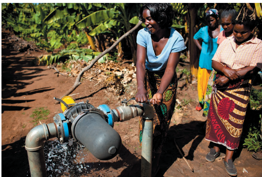
A hydro-powered irrigation pump in use at the Kabwadu Women's Banana Farm in Zambia.
