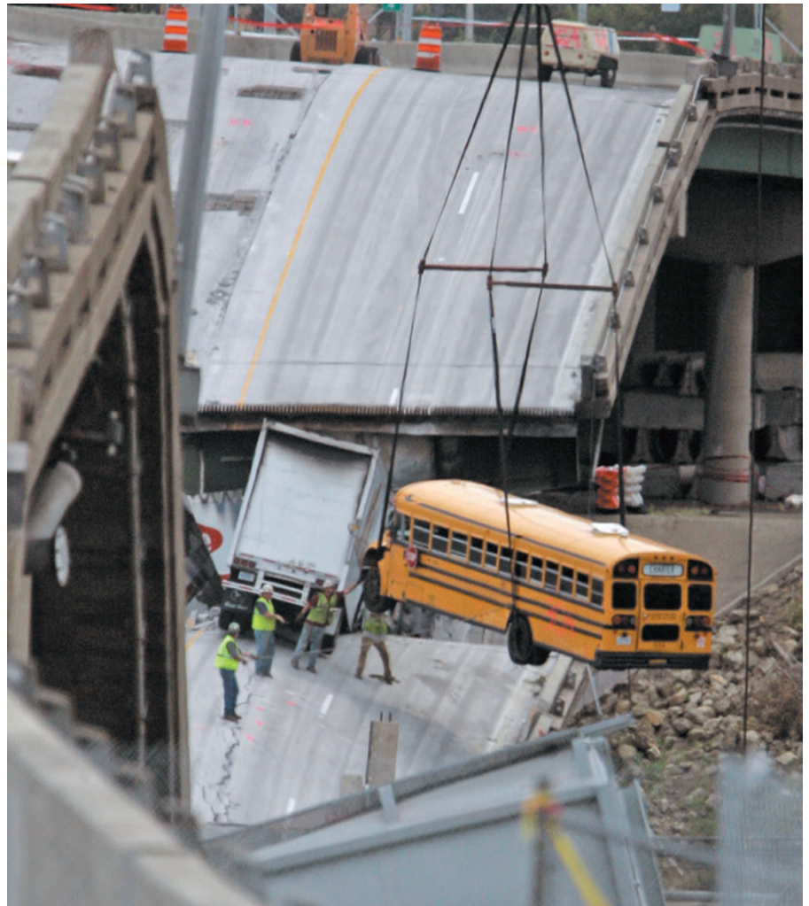
The heavily used I-35W bridge in Minneapolis, Minnesota, collapsed in 2007.
