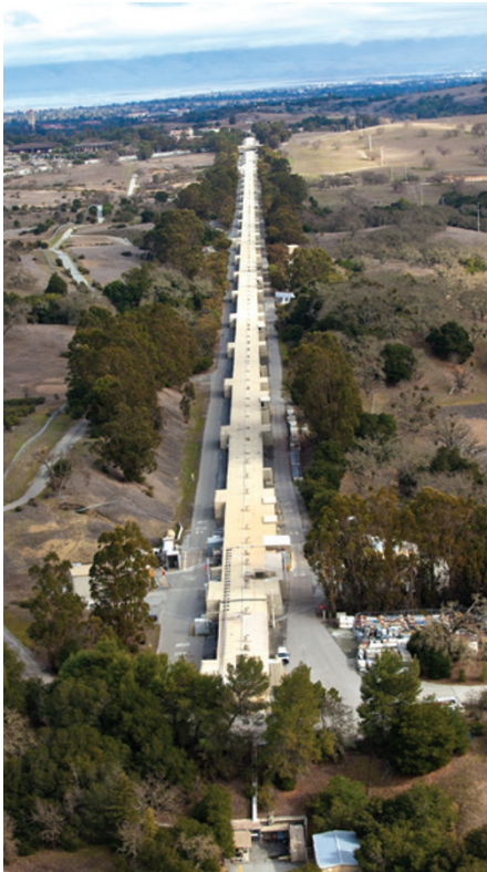
Stanford's SLAC relies on 284 microwave pulse generators in its particle accelerator, which is more than three kilometres long.
