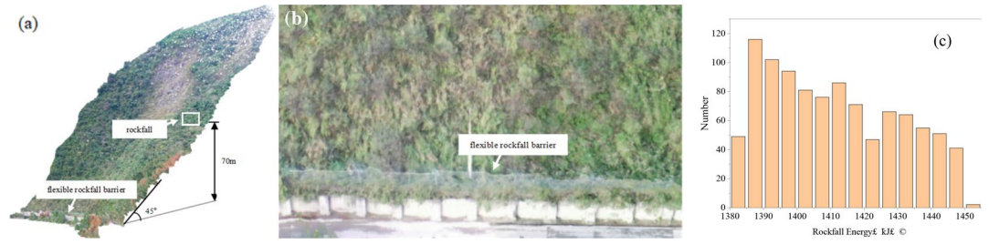
Figure 13. Locations of the rockfall sources and the flexible barrier.
