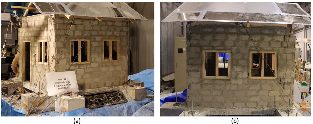
Figure 3. Cracks pattern of the non-retrofitted house model after run 34. (a) Out-of-plane failure on the north and south walls, (b) in-plane failure on the east and west walls.
